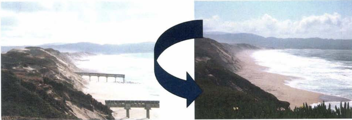
Storm drainage outfall removal – Before and After
